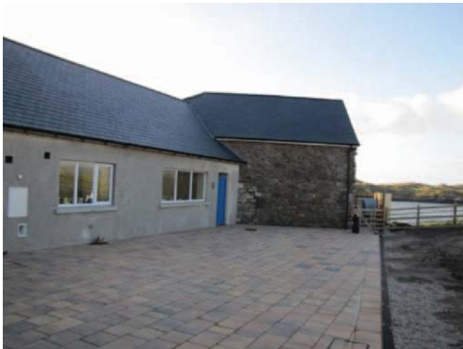
Figure 19: Lime render finish, heat pump at rear
