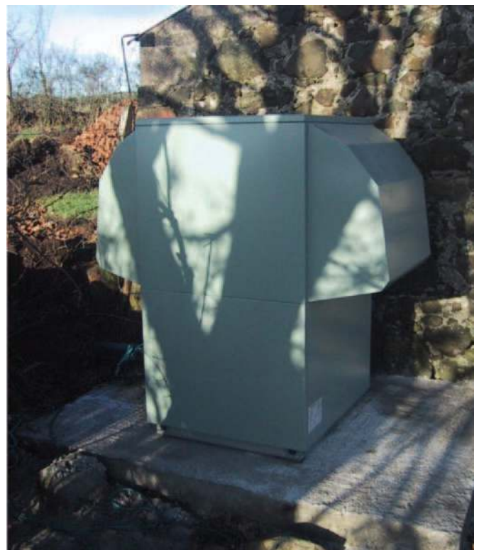
Figure 5: 16kW single unit ASHP (image courtesy of Element Consultants Ltd)
